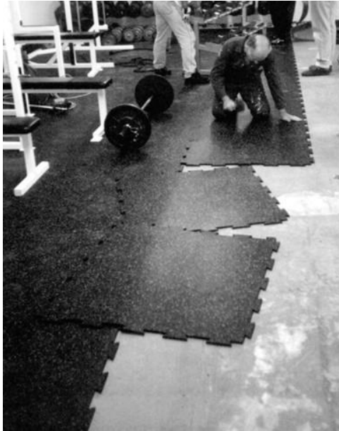
Four-Side Interlock Loose Lay Installation
